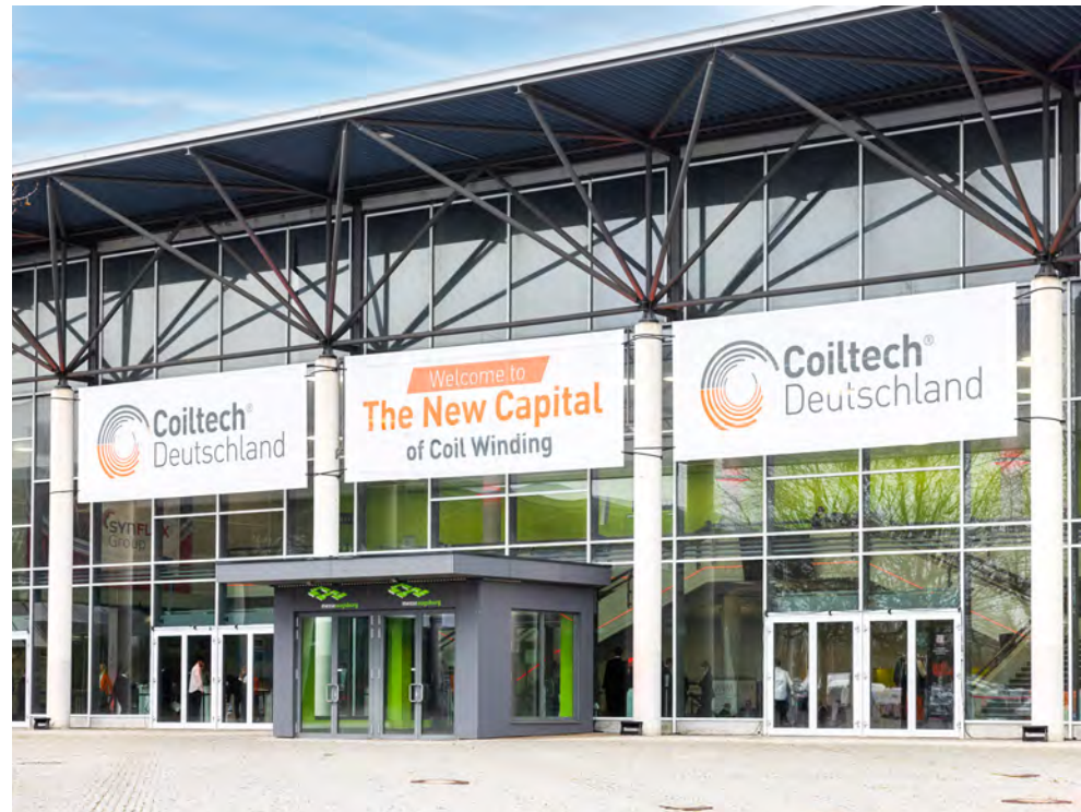
Fig. 1 – Banners in front of the glass façade / entrance area (outside)
